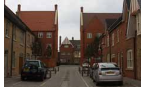
Simple roof shapes used to add interest to the street scene
