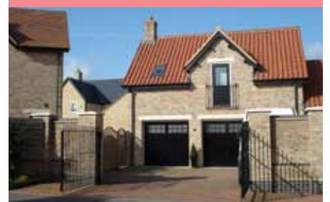
Gable end chimney on the ridge line
