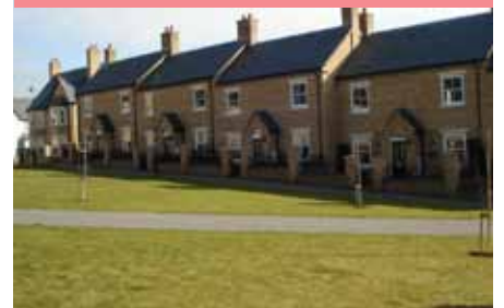
Simple slate roof steps down the terrace
