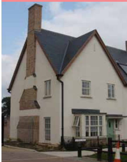
Architectural detail used on corner buildings adds interest and aids legibility
