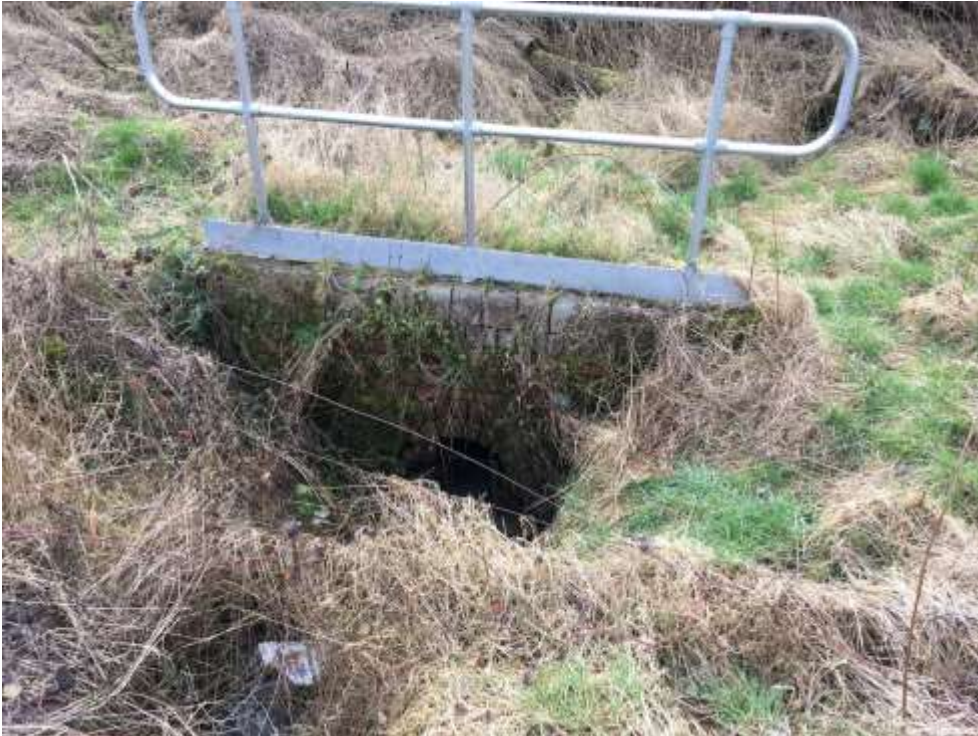
Figure 3.7 : Existing Watercourse 2 culvert under railway
