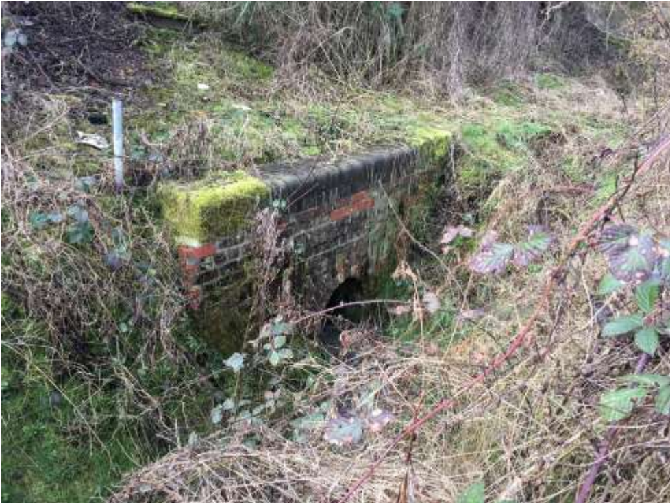
Figure 3.3 : Existing watercourse 1 upstream end of railway culvert
