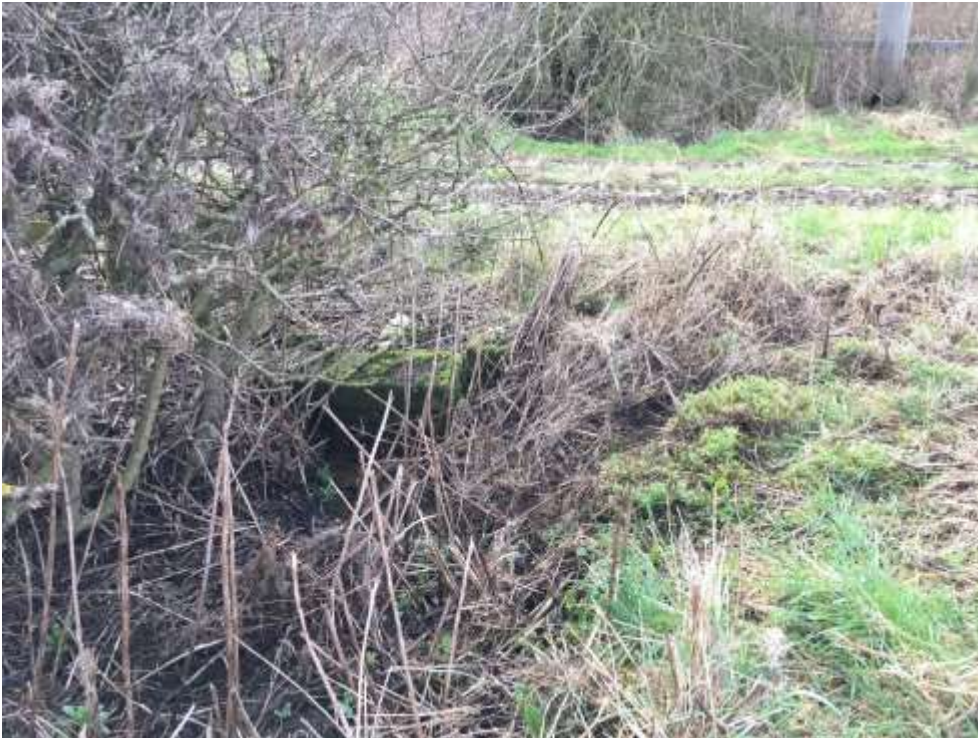
Figure 3.2 : Existing Watercourse 1 piped under farm access track
